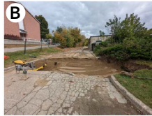
A - Exterior - View northeast
